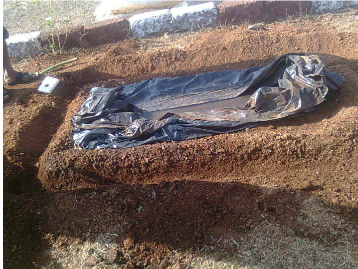
Plate: 2. Basin prepared in soil for W-shape solar still on soil
