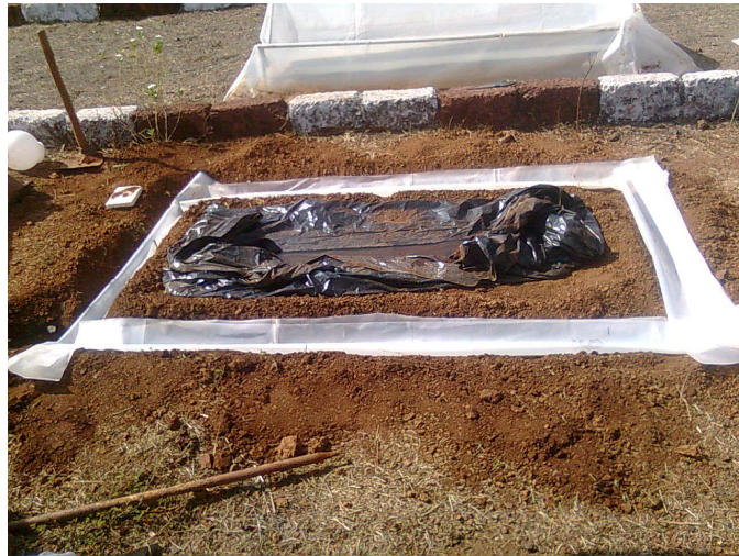
Plate: 3. Third channel from all bottom sides for W-shape solar still on ground
